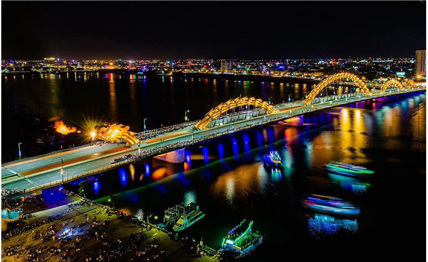
Dragon Bridge - Danang
